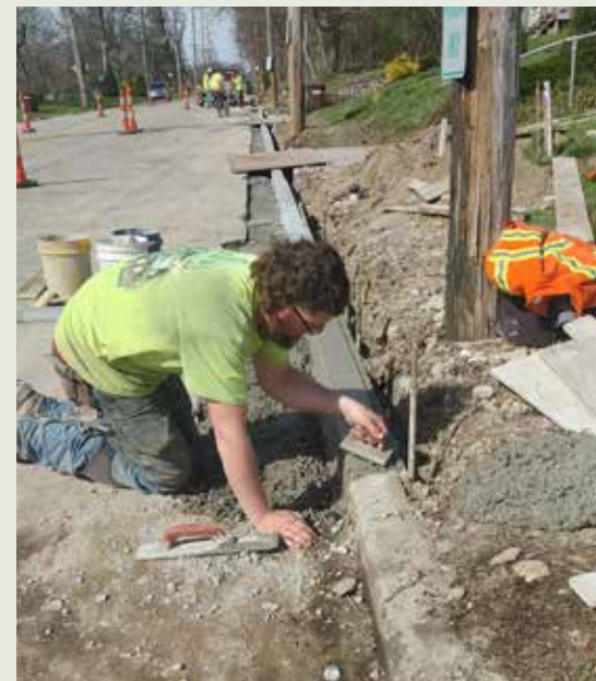
Curb work on Sutton Road is started before new sidewalks are constructed.
